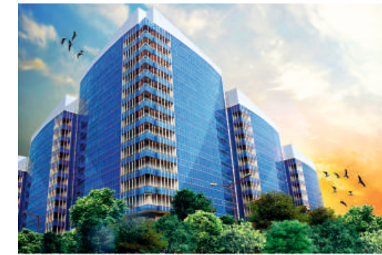
ANANT RAJ TECH PARK, MANESAR FIRST OPERATIONAL DATA CENTER
